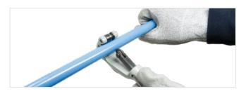
Prepare the tube for assembly. If necessary, cut the pipe using the appropriate FPTT tool. The pipe cut must be perpendicular to its axis (90  $^{\circ}$  cut).
