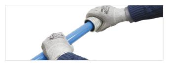
Always deburr the pipe, externally and internally, eliminating sharp edges, before making the connection with the fittings. Use the FPUS accessory.
